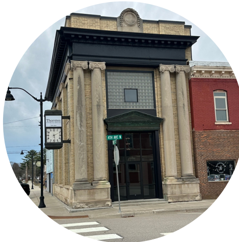
Facade improvements completed at 201 4 th Ave. N., Foley
